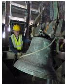
The bells are sent to Whitechapel Bell Foundry to remove the canons (old-style fixing points on top of bells), send them off to be sandblasted clean of corrosion, and then skilfully re-tune each bell. The bells continue their journey to Nicholson's in Bridport, Dorset to be assembled in the newly fabricated frame.
